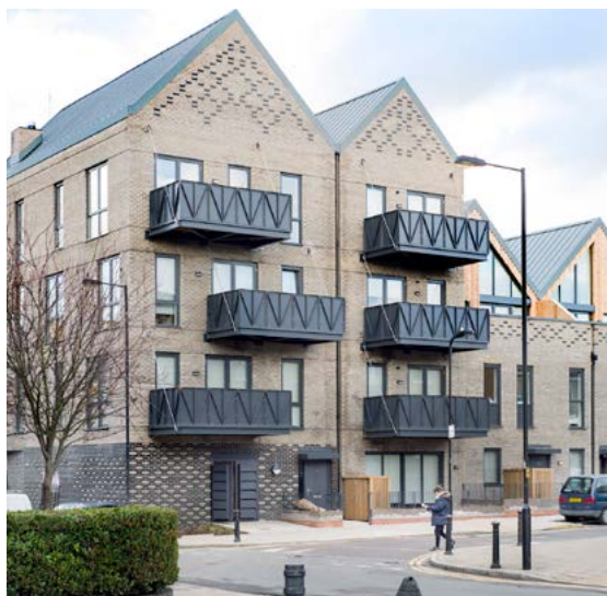
King Edward Road Estate, Hackney
